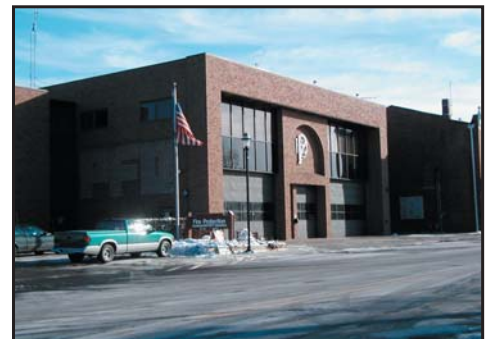
Plainfield Fire District Main Station
