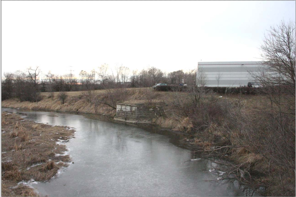
Above: One historic limestone bridge abutment exists along the DuPage River just west of Illinois Route 59 north of downtown Plainfield. The road originally curved to the west to cross the river more nearly perpendicular; the road was straightened to its present-day alignment in the 1930s. Below: The Spring Banks bridge at Renwick Road at the DuPage River is the only known steel truss type bridge in the survey area. It was constructed circa 1912 and is listed as a Will County Landmark.
